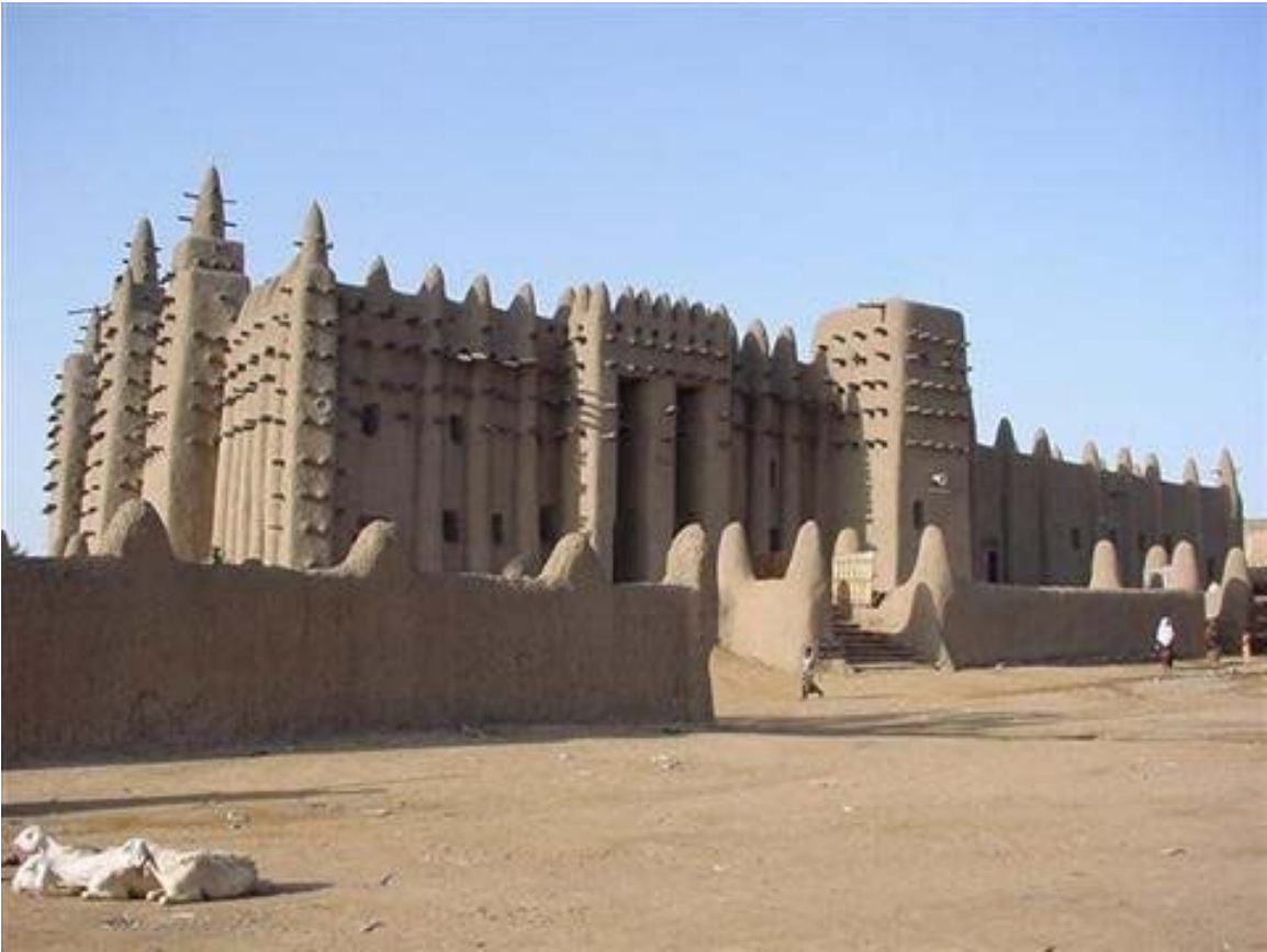
Mosque at Djenne
